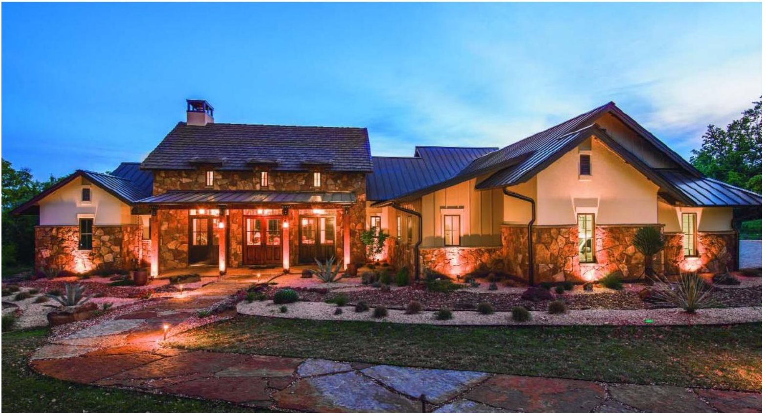
The house is designed with large overhangs that allow light to stream through the windows – but without the intense heat or cold.
